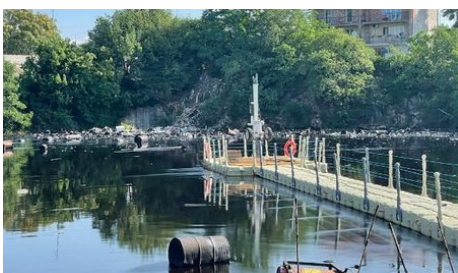
Pontile in acque oleose e acide con trivella per carotaggio Dock in oily and acidic water with core-drilling rig
