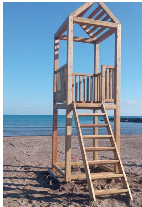
Torretta a 2 falde, in fase di montaggio Double-pitch tower during assembly
